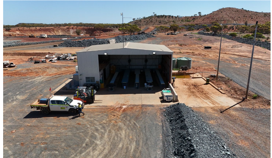
Figure 15 - Sand King – on site core processing facility
