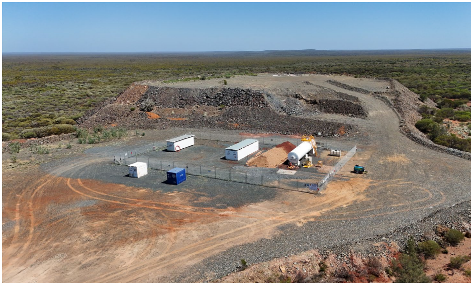
Figure 16 - Explosive and emulsion magazine
