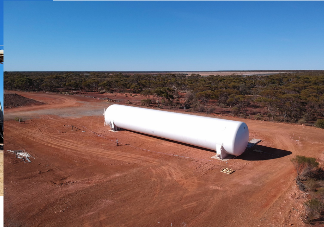
LNG tank for new power station in position
