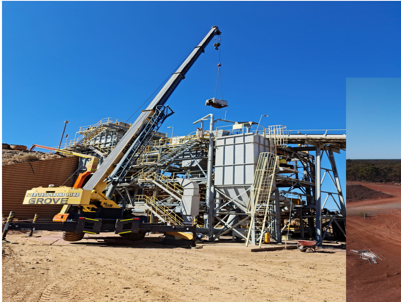
Installing conveyor head chute at crusher station
