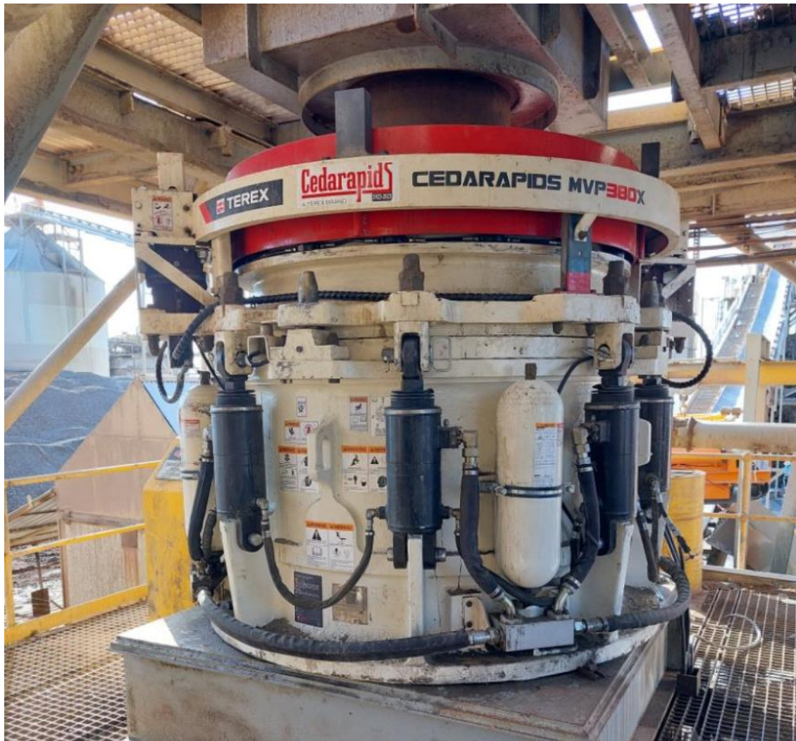
Figure 7 - New Terex 380 tertiary crusher installed
