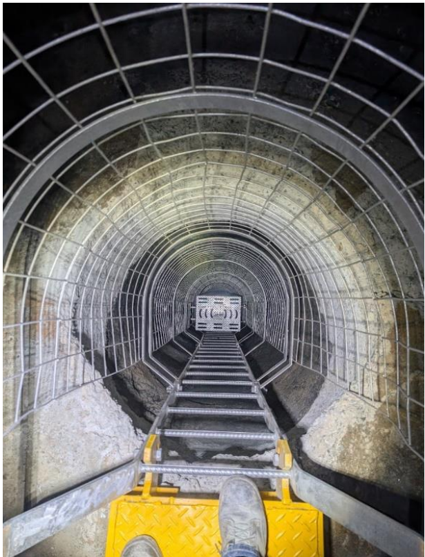
Secondary Escapeway (ladderway looking down)
