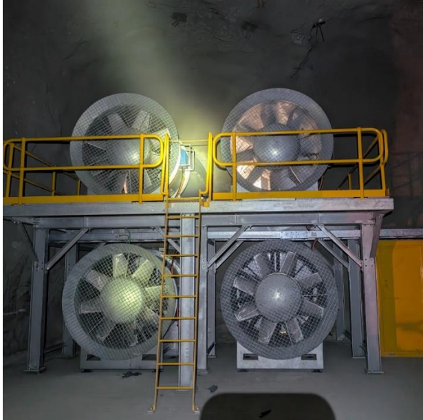
Primary fan installation
